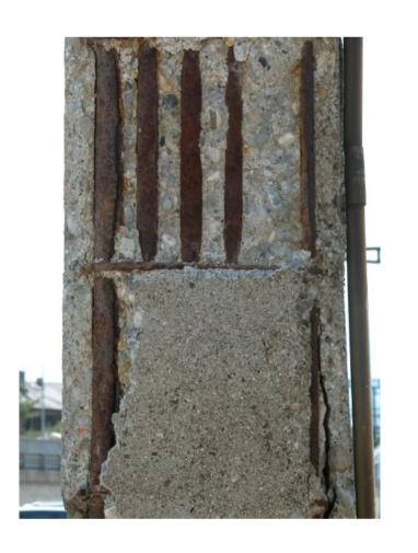
Chloride ingress is one of the main degradation process of reinforcement concrete. Source of chlorides include seawater or de-icing salts.
